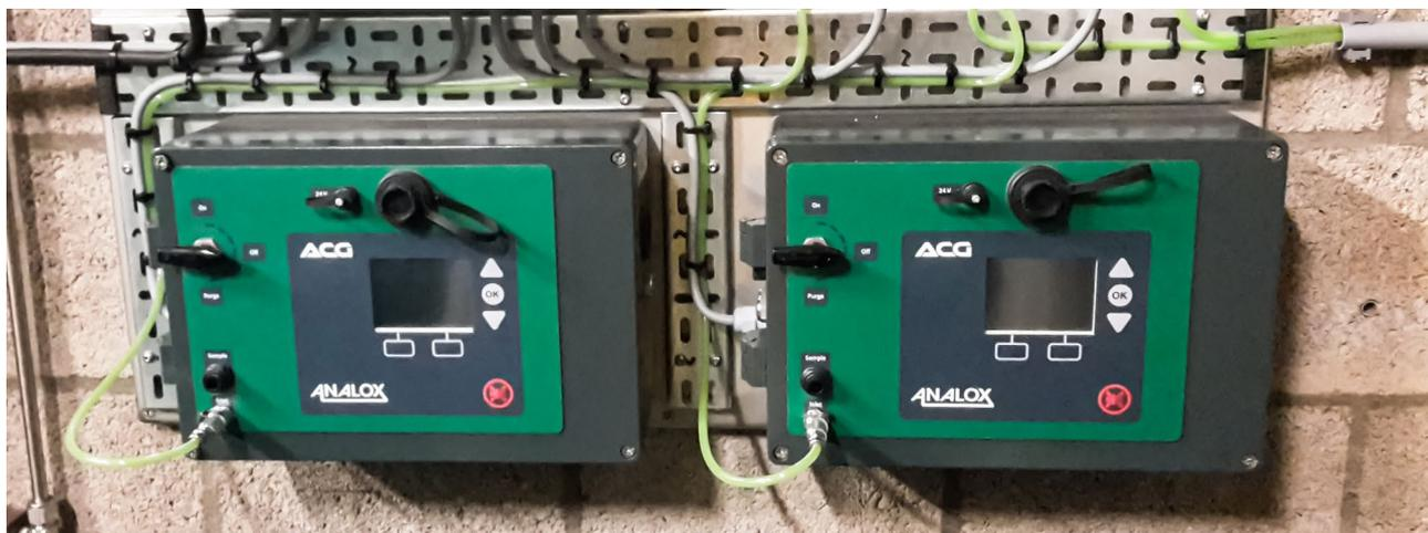
Both of the ACG units (image above) are fitted working on the **RNN diving simulator** for the air supply, ensuring the team controls the air out of the compressors. The ACG+ warns the team should any contaminants be detected in the breathing air supplied from the compressor.
